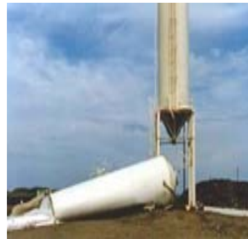
Figure A.2. Failure of grain silo.
