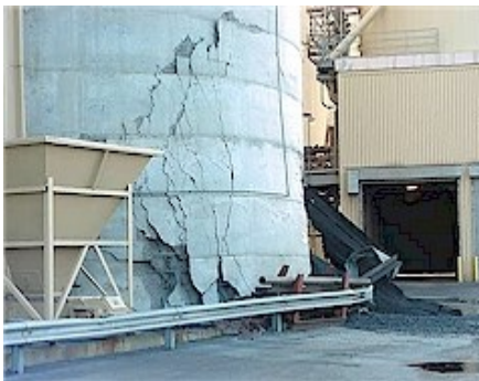
Figure A.5. A hole in a 12.7 mm thick stainless steel plate and a movement of a 2000 ton silo by shearing its foundation bolts, the USA.
