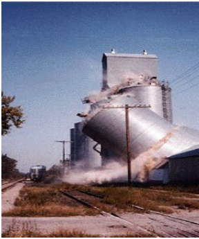
Figure A.3. Collapse of a granular (corn) silo due to a poor design.
